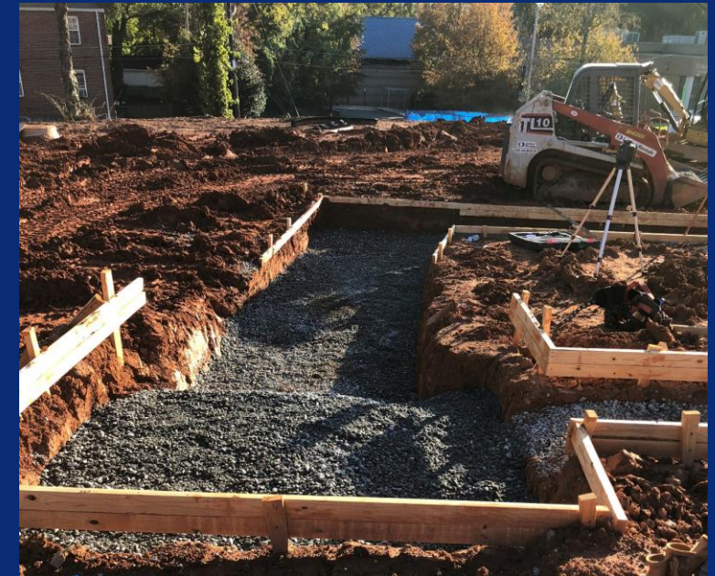
Prep for footings at main level east
