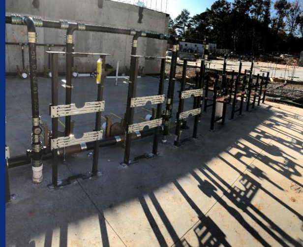
Carriers set in lower level restrooms
